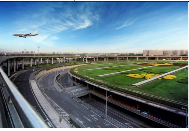
The landscaped green roof at Beijing airport.
